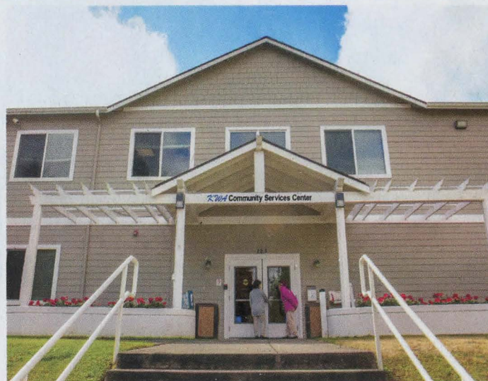
The KWA Community Services Center is located in Tacoma.
