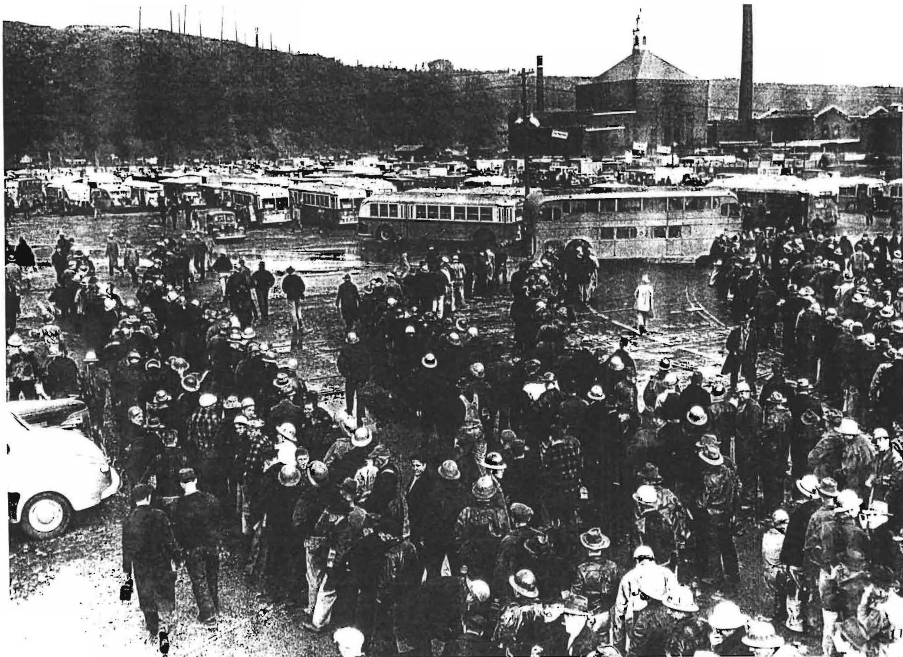
WITH GAS RATIONING DURING WORLD WAR II, MANY WORKERS RODE THE BUS TO THE SEATTLE-TACOMA SHIPYARD. (Richards Collection, Tacoma Public Library) For Tacoma, the war boom began in September 1939 when the U.S. Maritime Commission awarded the Seattle-Tacoma Shipbuilding Corporation a contract to build five freighters at a cost of $2,127,000 each. Thousands of people from the Midwest flocked to Tacoma to work in the shipyard. (F-4)
