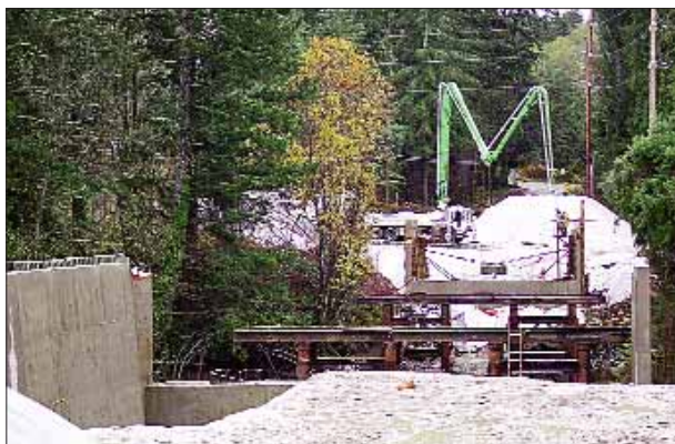
Vaughn Bridge Dec. 09
