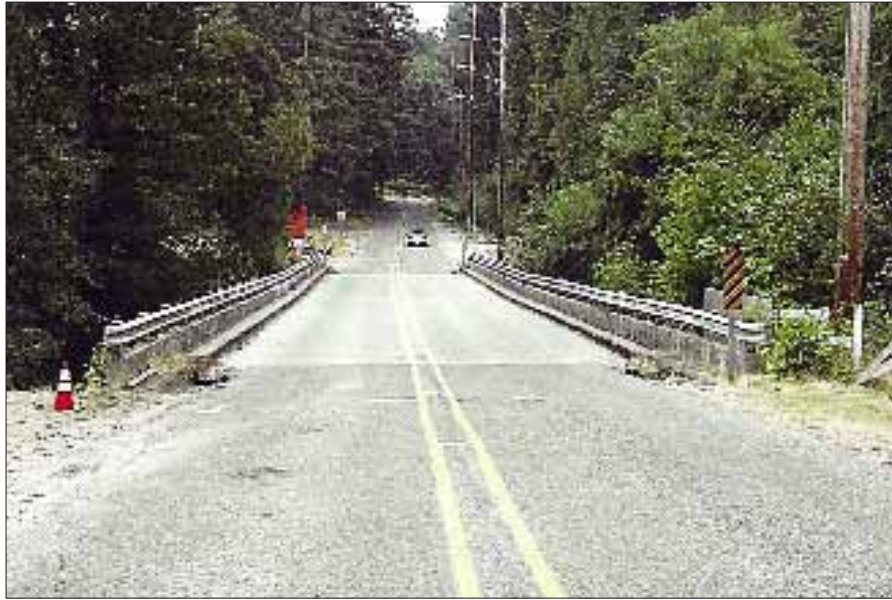
Concrete bridge built 1966
