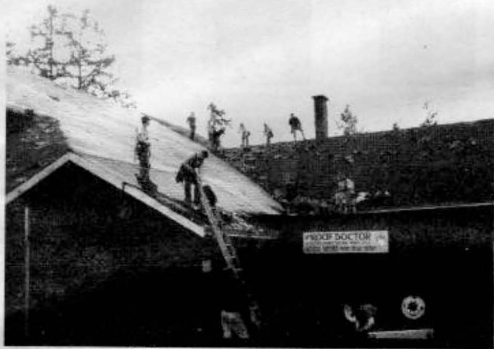
Workers putting new roof on Civic Center.
