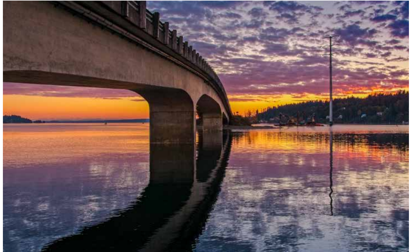
The Burley Lagoon project, which includes new transmission lines and one taller tower that replaced the four 1926 towers, is an improvement for the PenLight system. The work was coordinated between Tacoma Power, its contractors and PenLight operations crews. The results will provide a much more resilient power supply for PenLight members on the Key Peninsula, especially in the event of big wind or ice storms and will withstand greater seismic shock if we have a big earthquake. Photo: Jim Bellamy
