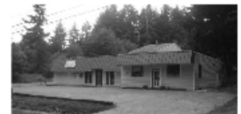
GIG HARBOR $475,000 What incredible opportunities this commercial property offers! Rent the commercial building, an opportunity to have 2 shops & rent out the large 2 story home in back or live in the house yourself & start your own business. The ideas are endless here! Cinda Baldwin 253-857-3304 #87888
