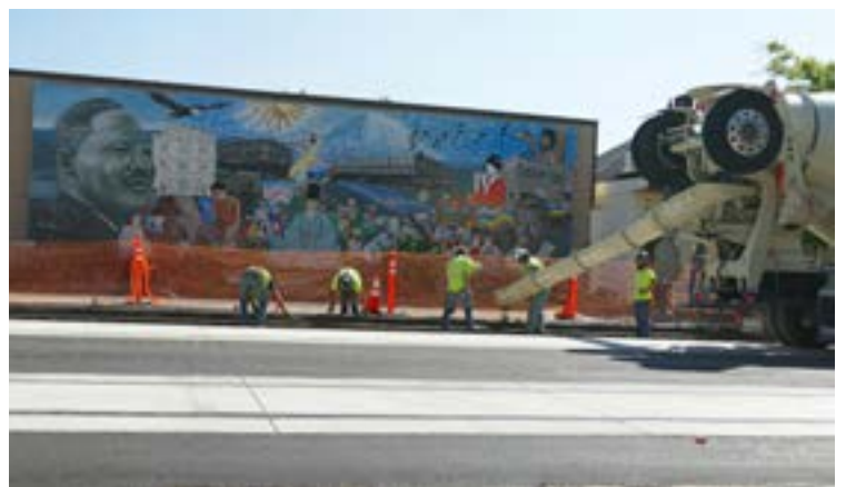
Pouring concrete for curb and gutter, Aug 4th
