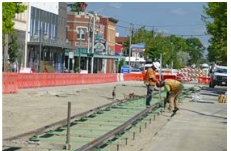
Preparing track on MLK Jr. Way south of 11 ST, Aug 4th
