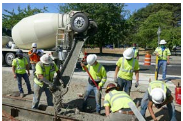
Crews pour concrete for curb on MLK Jr. Way, Aug 4th
