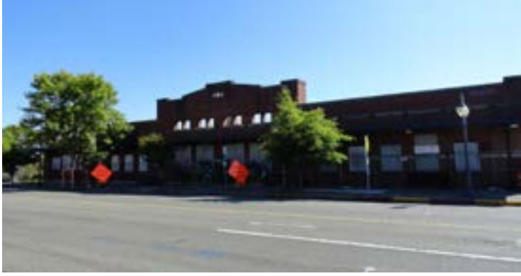
The Rite Aid site sits empty as a sign of community disinvestment. Forterra seeks to turn this perception around by listening and acting on what community members need from this space.
