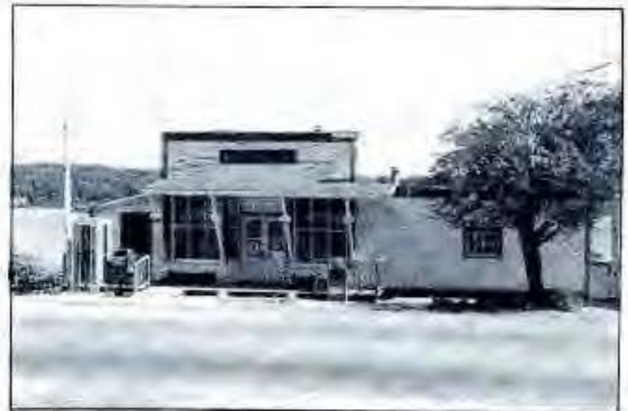
Wauna Post Office at the Purdy Spit ... due for a new location? KP NEWS photo by Lee Siles
