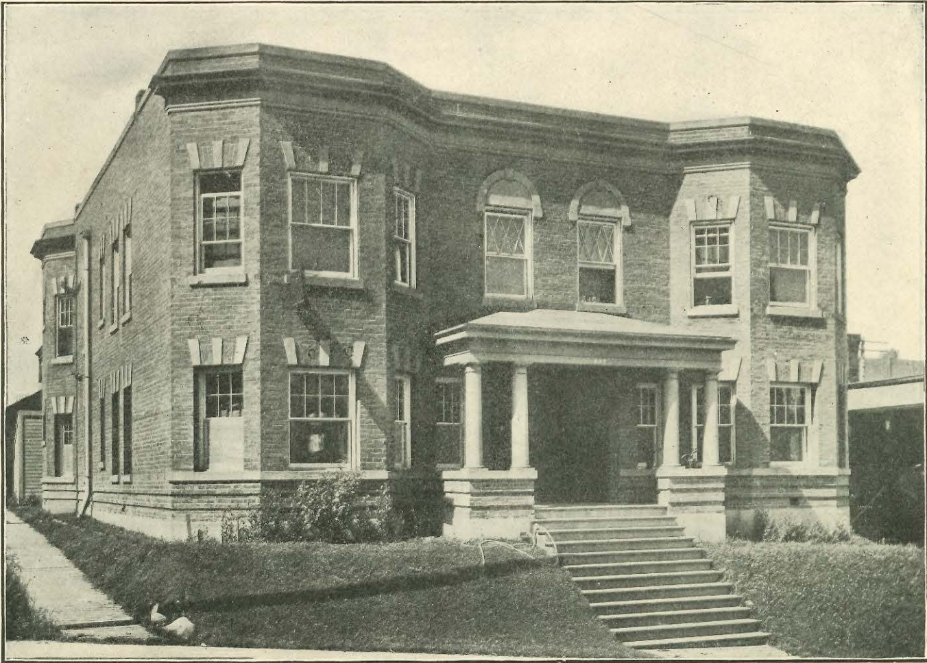
APARTMENT HOUSE ON SOUTH TENTH STREET, NEAR TACOMA AVENUE Russell & Babcock, Architects
