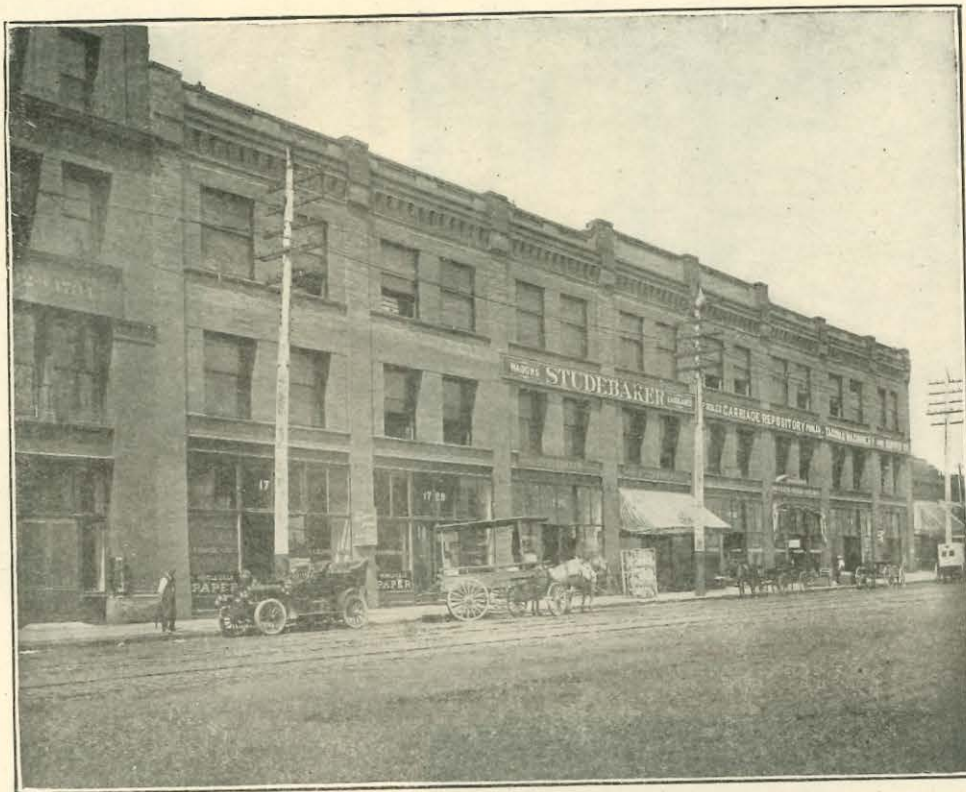
WHOLESALE HOUSES ON LOWER PACIFIC AVENUE Russell & Babcock, Architects
