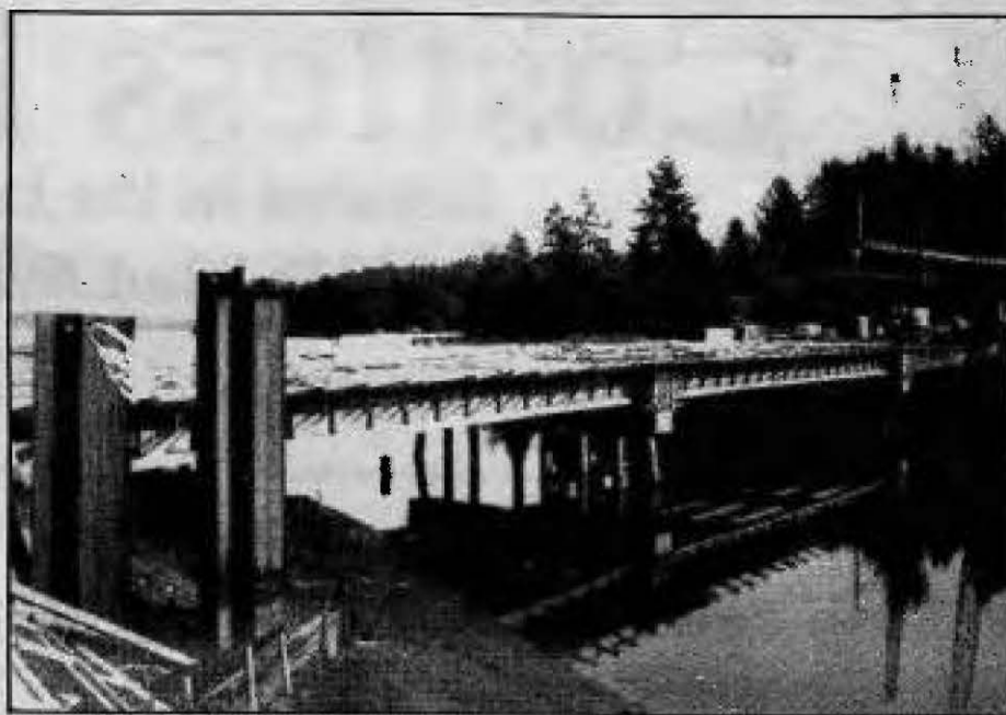
Work on the Home Bridge progresses on schedule. The enormous prefabricated steel-reinforced girders which will hold the roadway have trundled down the Key Peninsula Highway and, recently, around the tortuous detour's tight curves, before being lifted into place by heavy duty cranes. The span should be open to after the first of the year. photo courtesy of Hugh McMillan
