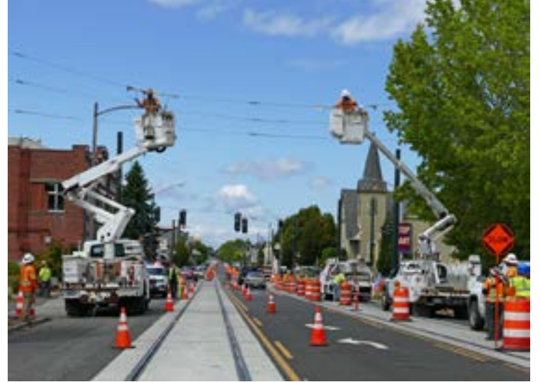
Hanging wire span above MLK north of 15th. Photos courtesy of Liz Ellis.
