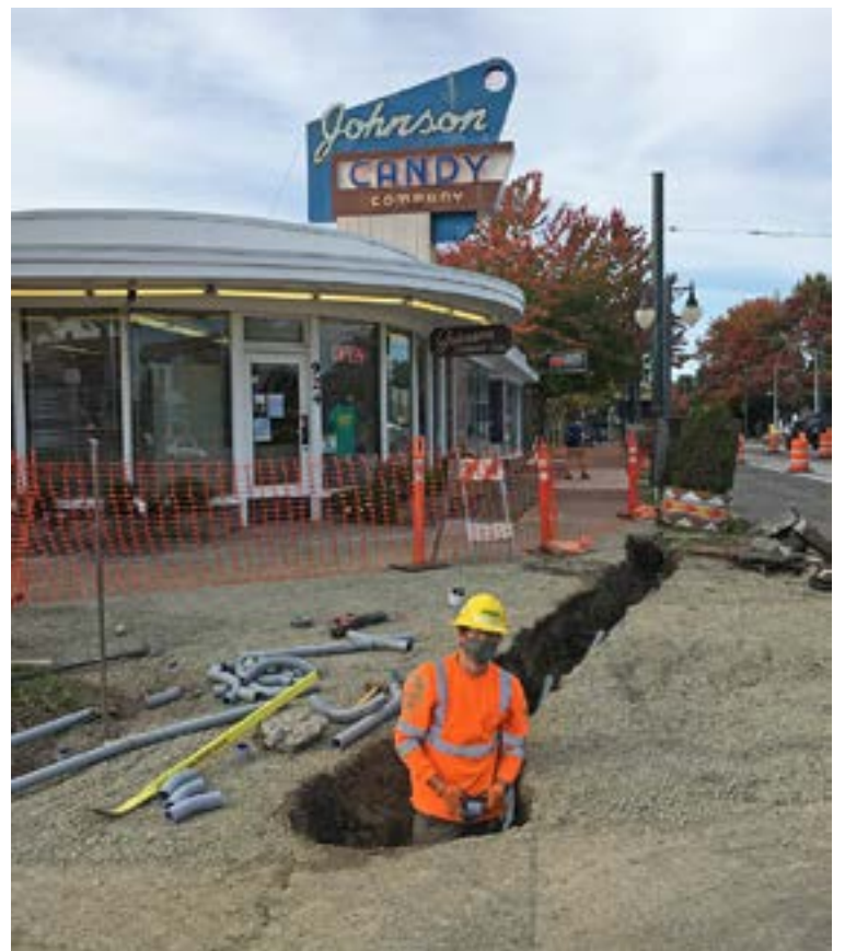
Conduit installation next to Johnson Candy Company.
