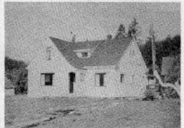
The "new" house after completion in 1935.
