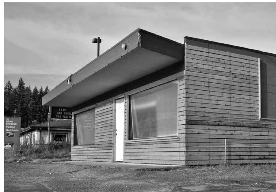
Owners begin to transform their acquisition into Madrona Cafe. Photo: David Zeigler, KP News
