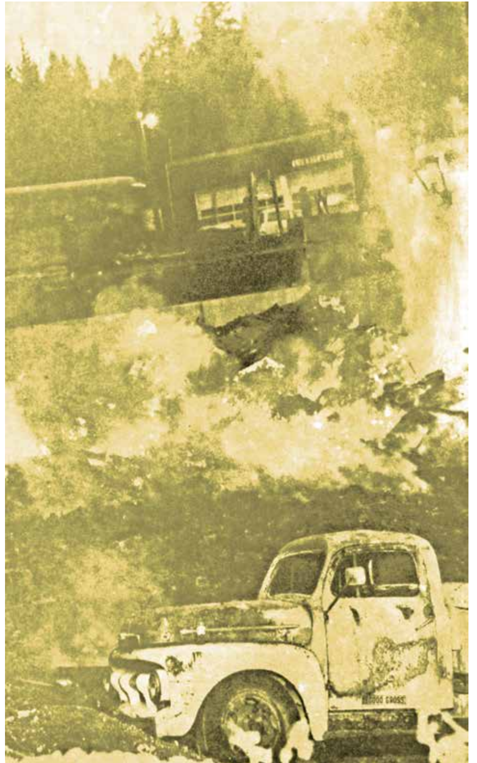
The scene of the fire in the early morning, looking up from the bottom of the gully towards the gas station across the intersection. Photo: Bob Boxberger, collection of Nadine Niemann.
