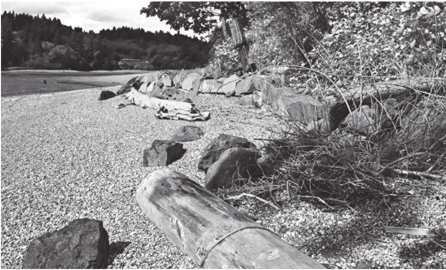
The Taylor Bay Community applied for a permit from Pierce County when it sought to protect the boat ramp on the community beach. Following recommended guidelines, the plan used natural armoring, including carefully placed logs anchored with stainless steel cable and gravel to help preserve habitat. Photo: Don Tjossem, KP News
