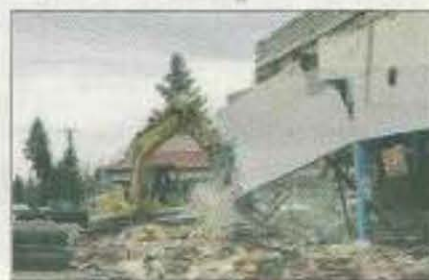
Peninsula Market demolition
