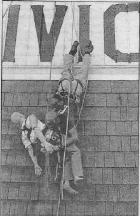
One of us is upside down and it isn't the sign.
