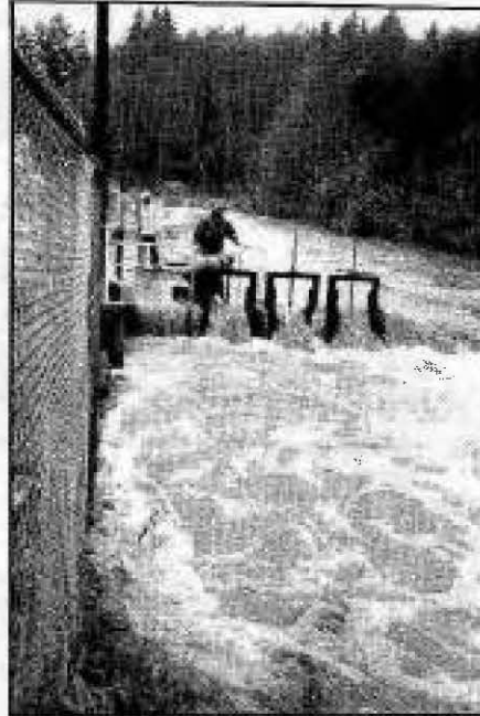
Flooding at Minter Creek Fish Hatchery. photo Hugh McMillan
