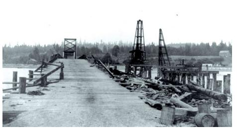
The third bridge under construction in 1920, south of the old bridge. Two pile drivers working on the new bridge can be seen on the right. This view is from Wauna looking east. *Harbor History Museum*
