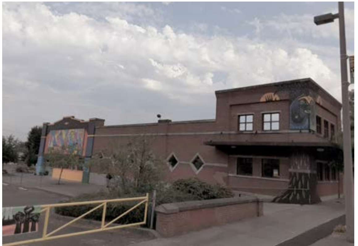
The Rite Aid building at the intersection of S 11th ST and MLK Jr. Way has been activated with local artist's murals. Forterra will transform this lot into an anticipated 300 homes and approximately 25,000 square feet of commercial space. Picture Courtesy of Kristine Coman.
