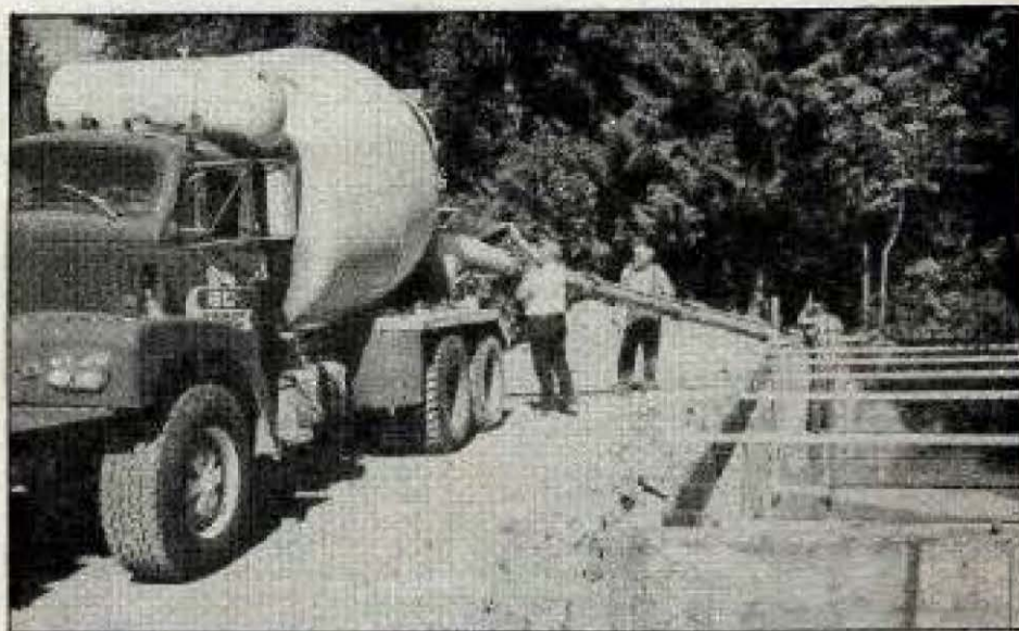
Gary Giuntoli from BoMac Gravel, Henry Stock and Lorrie Jopp pour concrete for the new Pioneer Days fishpond.
