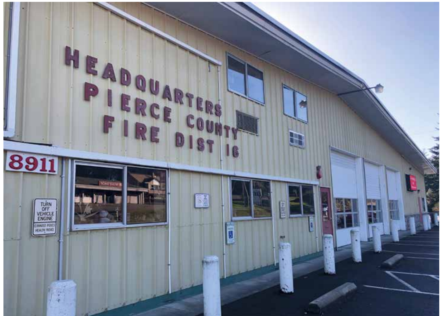
The fate of Station 46 in Key Center remains an open question in the budget. Ted Olinger, KP News
