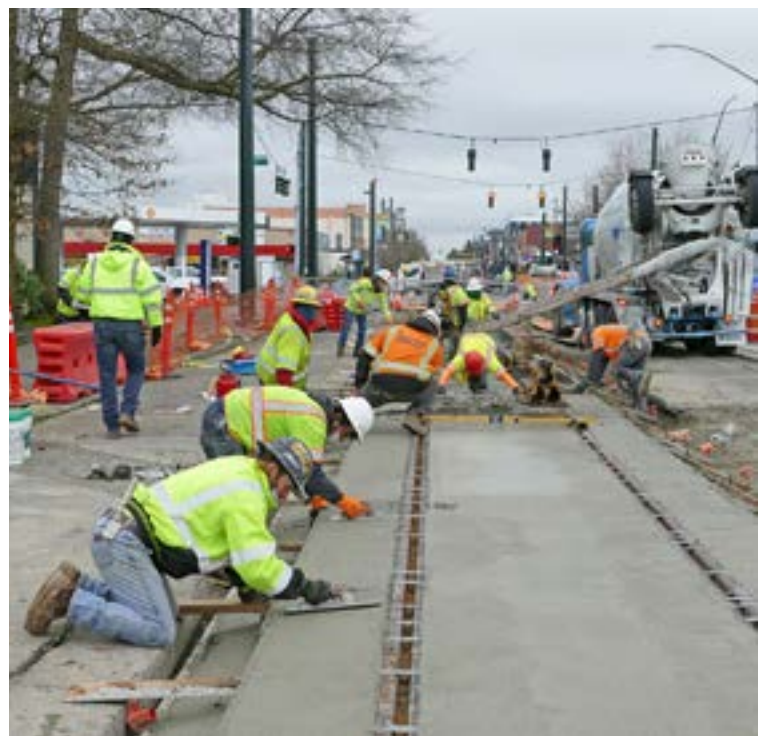
This photographs show the concrete pour around the tracks on Martin Luther King Jr. Way between South 9th Street and South 7th Street in March. Below are photos of 2 sets of tracks on Martin Luther King Jr. Way.
