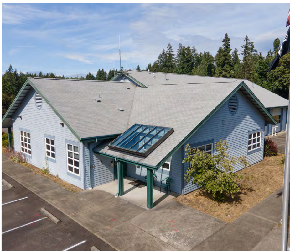
Longbranch Fire Station No. 49 is ready for occupancy. Photos: Caleb Galbreath, KP News
