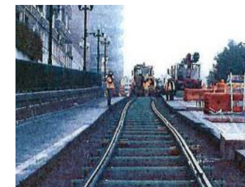
Grade & Move Rail into Place
