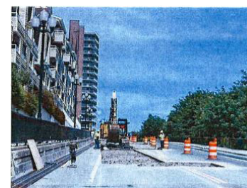
Remove Asphalt & Soil
